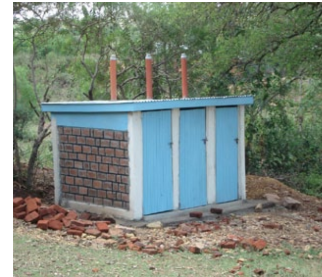
Figure 17: Ventilated improved pit.
