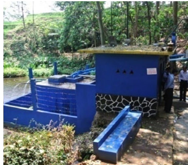
Figure 10: A community-managed water supply system in Malang, Indonesia
